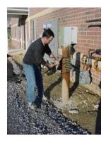
**Step 4** – Apply the material at the optimum height for vehicle protection and visibility. Multiple layers of 12" Bumperwrap™ can be applied to achieve 24" or more of protection.
